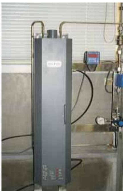
Fig. 3.2-5 Gas purifier (Ultra purity Purifier)
