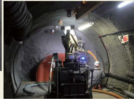
Backfilling test by spraying method
